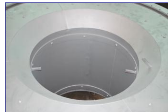
Eliminated structural ribs and associated welds
